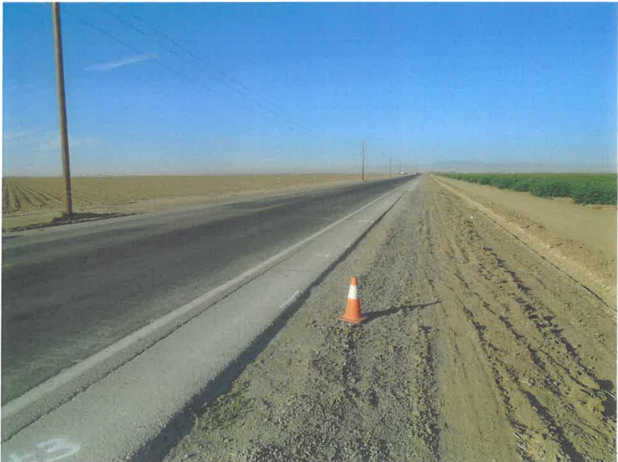
Near Boring B103 looking southwest.
