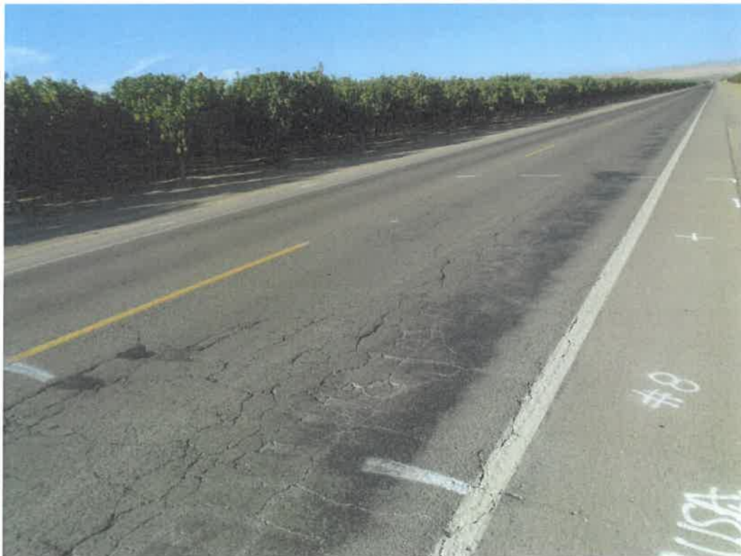
Near Boring B108 looking southwest.
