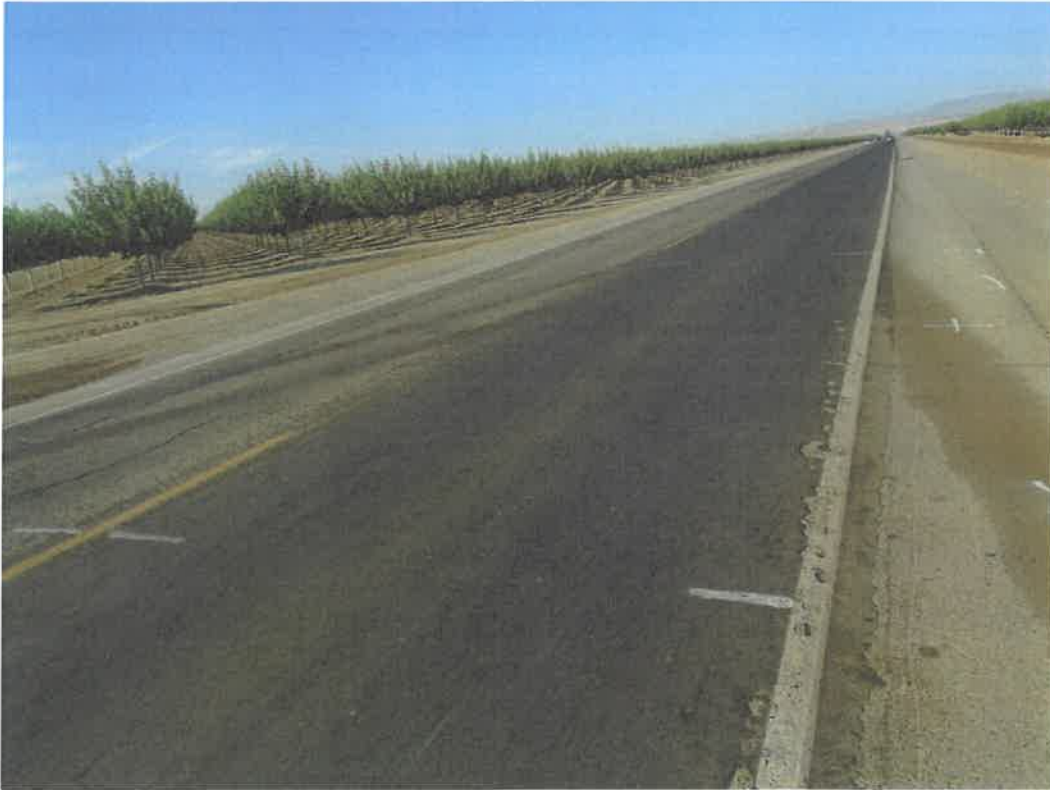
Near Boring B106 looking southwest.
