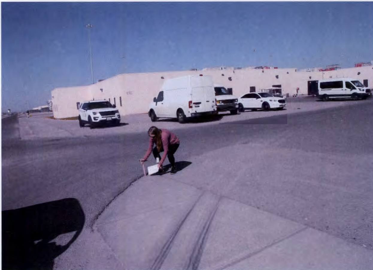
Effective 5/21/2020 repairs were completed.
