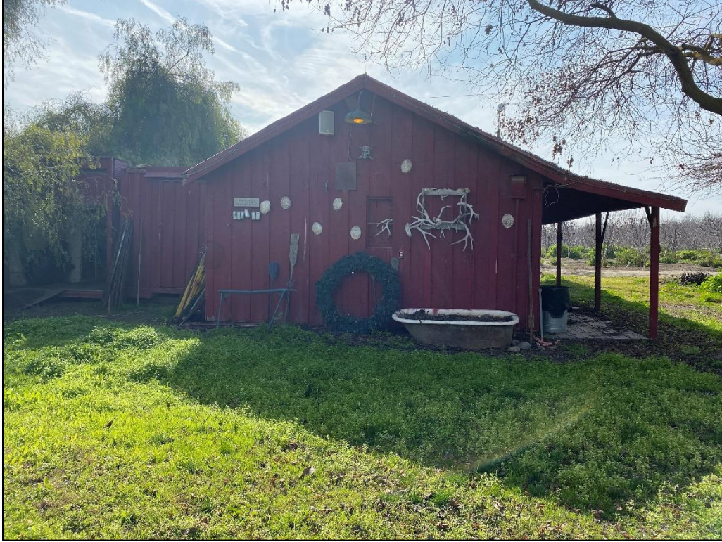
Figure 4-3 Northwestern portion of project site, facing south. Outbuilding in foreground.
