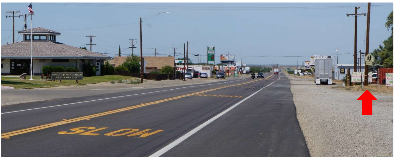
Figure 1 - Northbound Advance Warning Signage
