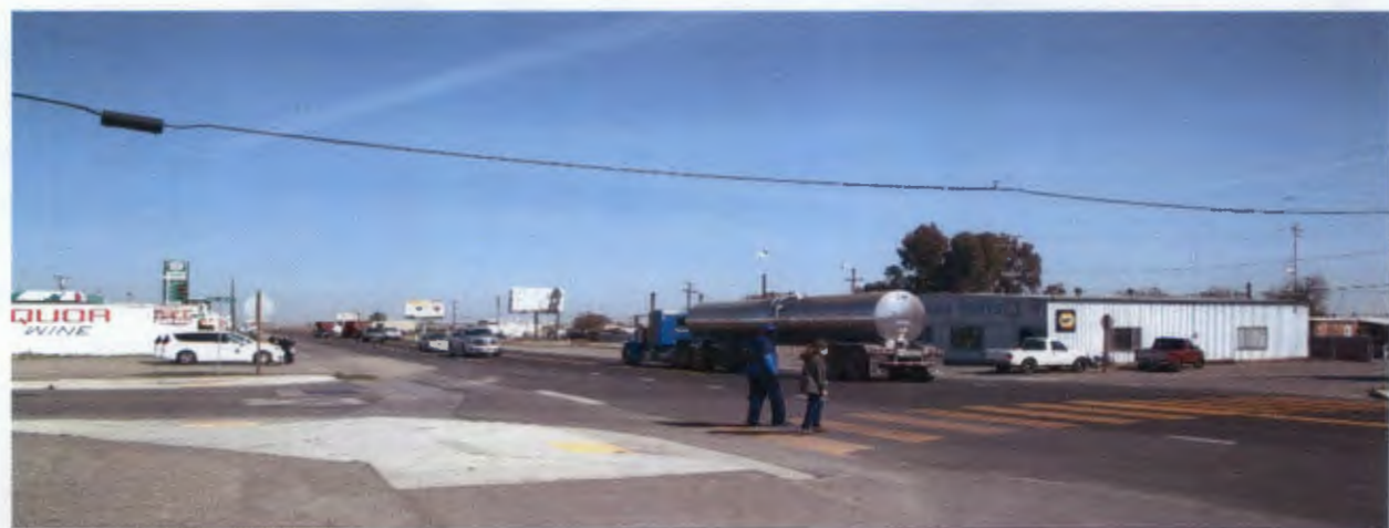
Figure 4 - Northbound View of Crosswalk
