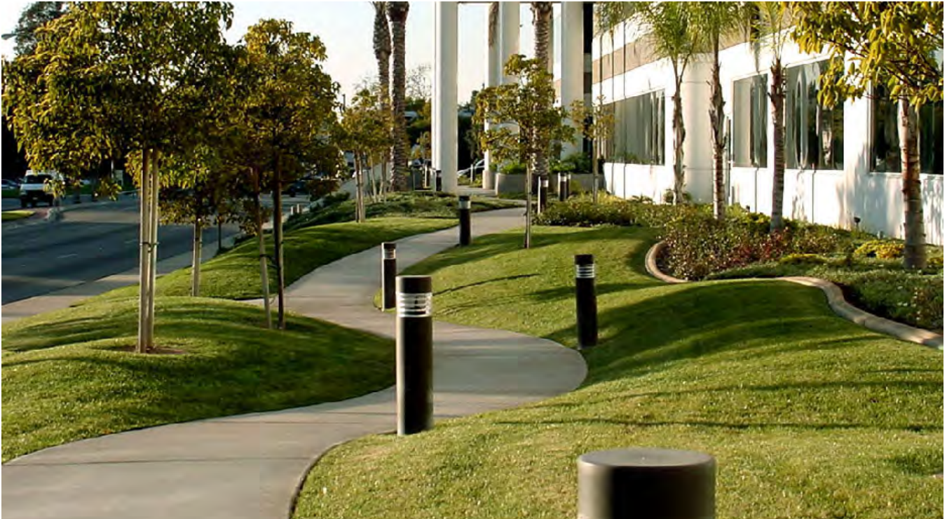
EXAMPLE OF BOLLARD LIGHTING ALONG A PRIVATE WALKWAY
