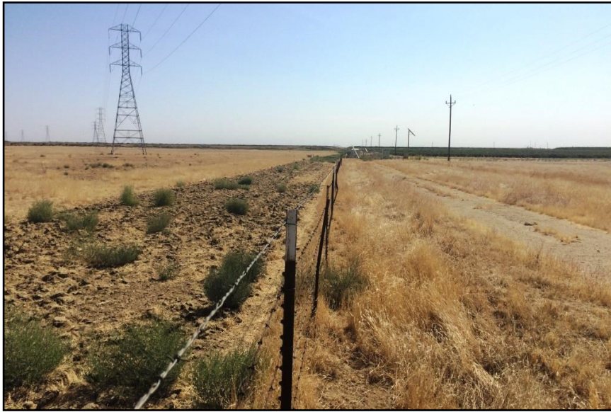
Photo 1. Southwest corner looking east along the south border of the project site
