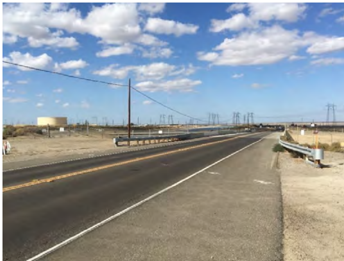
SR 41 at Aqueduct Crossing
