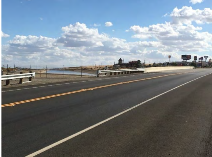
SR 41 as it crosses the aqueduct
