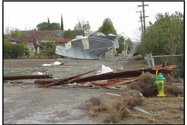
Figure HS – 10 Wind Damage in Avenal 2008
