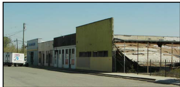
Figure 4.1. Existing deteriorated buildings
