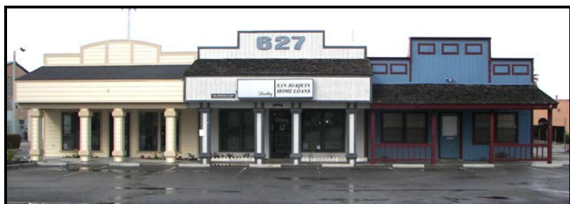
Figure 4.5. Commercial western facade example with overhang
