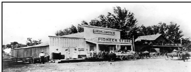
Figure 2.3. Kingston Historic Buildings 1870
