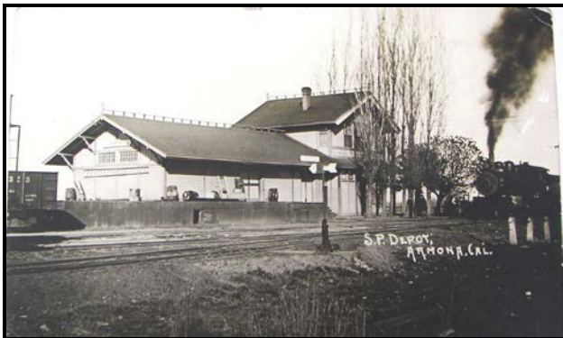
Armona Depot 1915 – looking northeast
